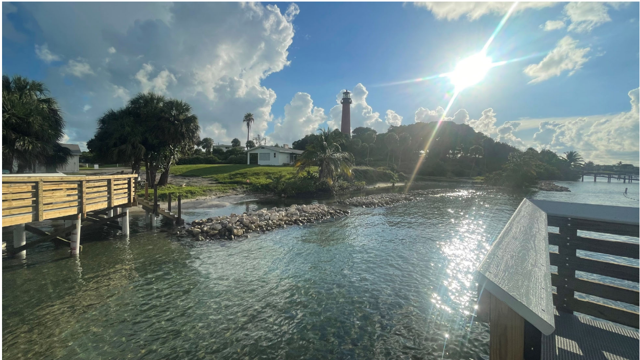
Photo 3-View of recently constructed living shoreline at the Jupiter Inlet Lighthouse Outstanding Natural Area
